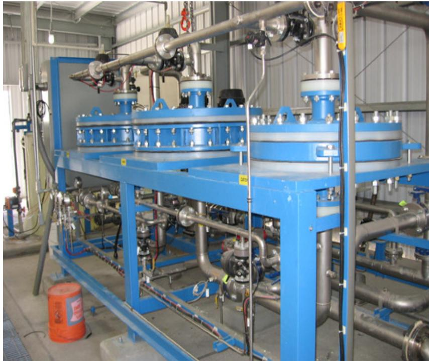
***Eco-Tec's compressed short bed Recoflo™ Triflo demineralizer/polisher Ion Exchange unit in a 1 x 100% configuration, at a generating station in Mexicali, Mexico.***
