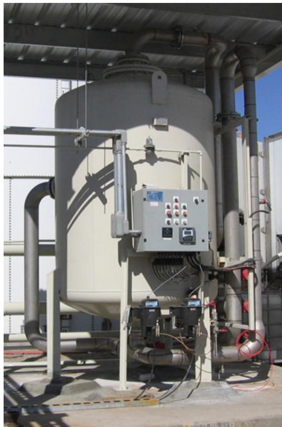
***Pretreatment using a single high-efficiency Spectrum Micro Media Filter™, which replaced four pre-existing sand filters.***
