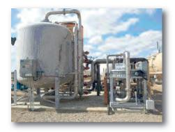
A 30,000 BPD Spectrum Plus Filter™ feeding an Eco-Tec RecoPur® SAC brine regenerated softener supplying a steam generator.
